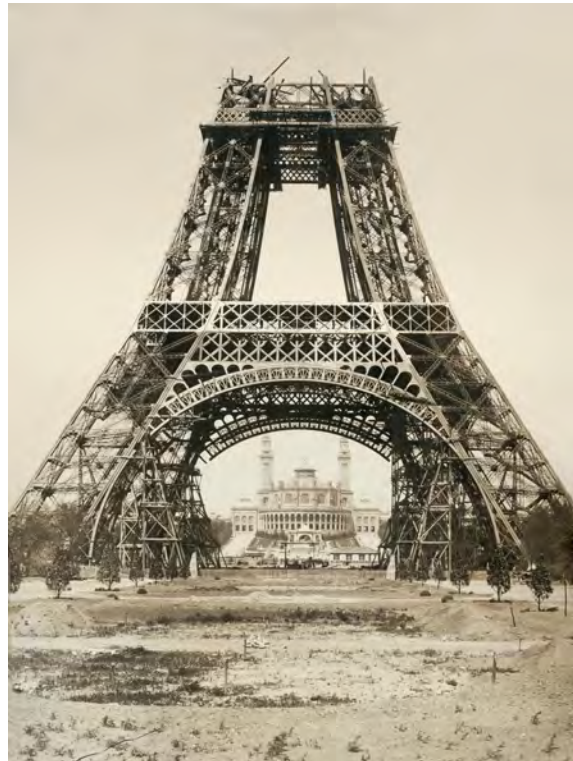
The Eiffel Tower under construction
