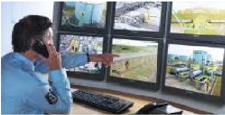
CCTV Monitoring System
