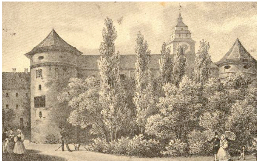
41 On the foundation of the Prus fortress Tuvangste in 1255 Konigsberg castle was erected by the Order as seen at the end of the XIX th century.
