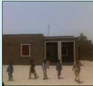
Construction of 4,500 One and Two Room Shelters/Houses 20,000 transitional shelters
