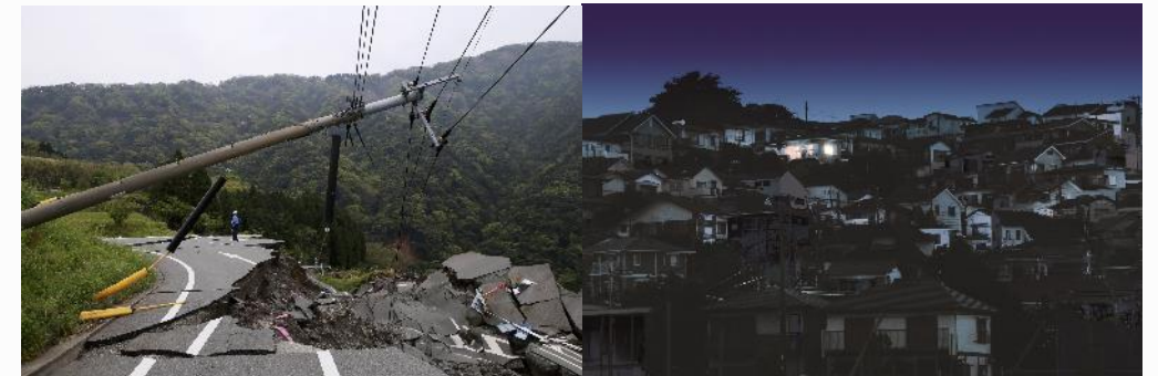
(Case) Damage to roads and power lines caused by earthquakes and large typhoons: prolonged large-scale power outages in urban areas
