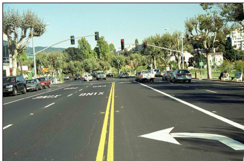
Typical left-turn pocket at a signalized intersection.
