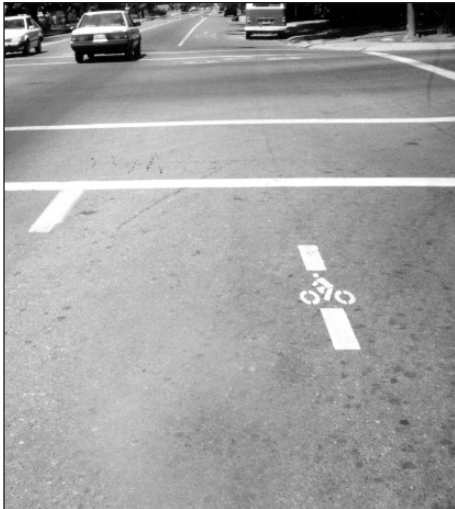
With no traffic to trip the detector, this loop detector pavement marking tells the bicyclist where to wait.
