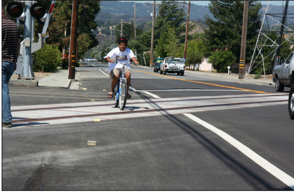
New concrete railroad crossing at Cox Avenue in Saratoga, funded by Measure B.
