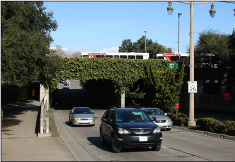
At University Avenue in Palo Alto, the wide sidewalks are higher than the roadway thereby reducing the grade change for both pedestrians and bicyclists.
