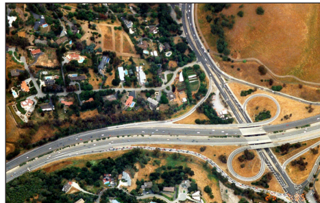
Typical Type L-9 freeway interchange of the 1960's designed with only motor vehicle traffic flow in mind; new and modified partial-cloverleaf interchanges should look like Figure 5-12 instead.
