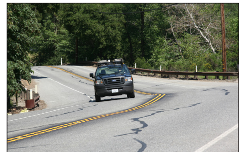
Centerline rumble strip on Highway 9 in Saratoga, where there is a wide shoulder.
