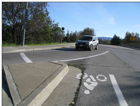
Even with a bike lane, these weave areas at freeway on-ramps are challenging due to the angle of the ramp departure from the roadway.
