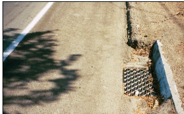
Recessed grate (WB Capitol Expwy near Seven Trees)
