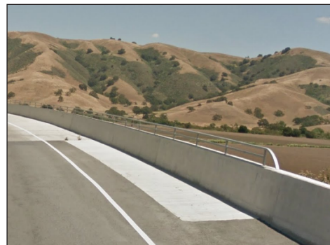
The S.R. 152 flyover of S.R. 156 adds a bicycle railing as it gains elevation. Since bicyclists will only be on the right hand shoulder, it is only needed on the right side of the flyover.
