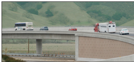
The new grade- separated overpass of eastbound SR 152 at SR 156.
