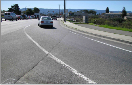
An approaching bicyclist would find himself to the left of this automobile entering from the cross street with a free right-turn lane.
