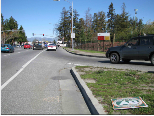
Free right-turn lanes at freeway off-ramps can be more problematic than at other locations due to the higher speed of traffic coming from the freeway.
