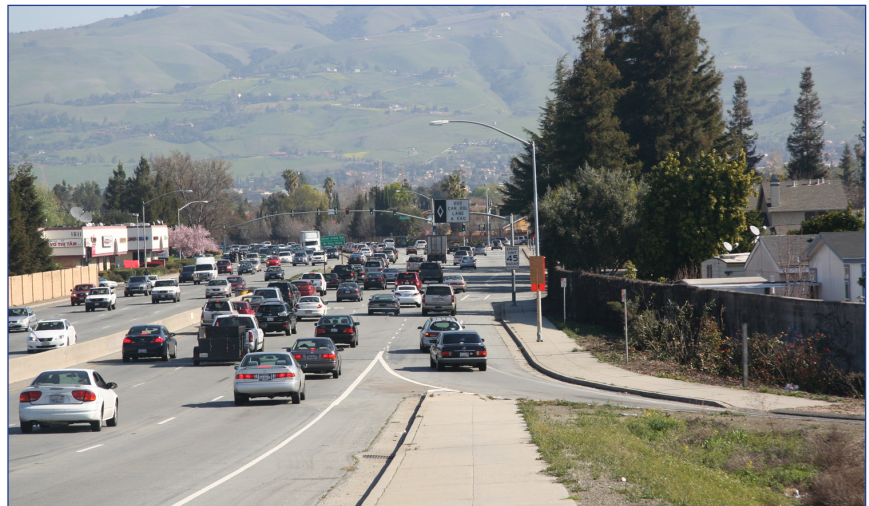
A through bicyclist will find himself in between two lanes of fast moving traffic at this location with a free right-turn lane.
