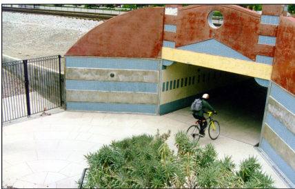
San Antonio Station Pedestrian/Bicycle Undercrossing of Caltrain tracks, Mountain View, opened 1988.
