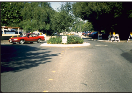
Residential traffic circles at two consecutive intersections provide better traffic calming effects.
