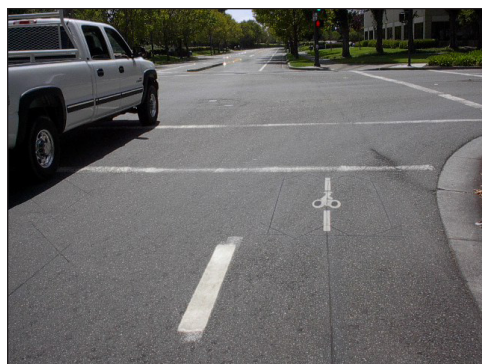
This Type Q detector in the bike lane means that the bicyclist will trip the signal without deviating from the normal travel path.
