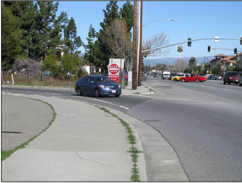
Pork-chop island designs often allow motorists to turn without stopping at the signal.
