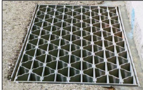
County Type 1C ("honeycomb") grate
