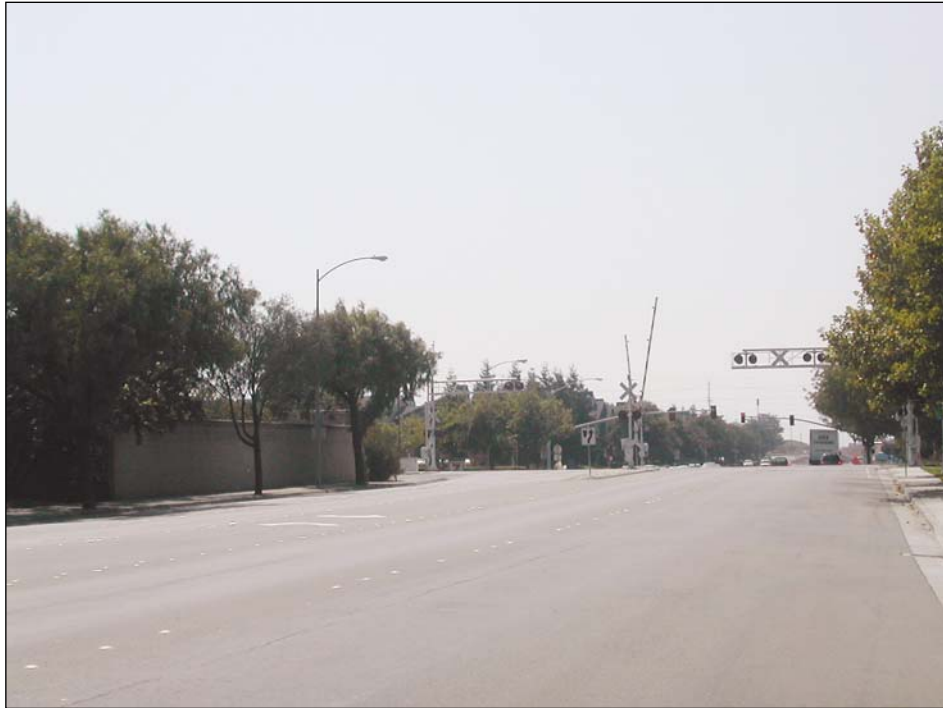
Figure 4.17-5: Dixon Landing Road (View to the west from Dixon Landing Road)
