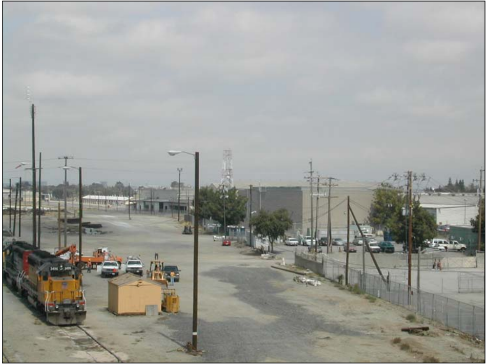
Figure 4.17-18: Maintenance Facility Location (View to the northwest from I-880)
