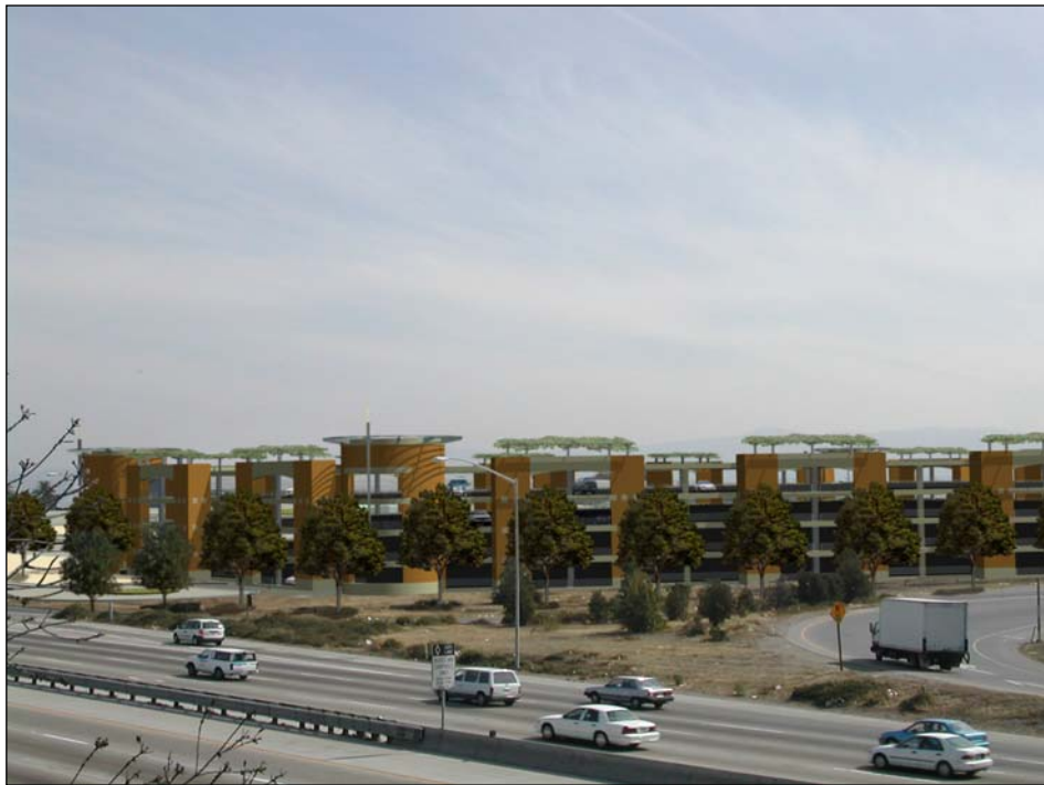
Figure 4.17-27: Alum Rock Parking Garage (View to the southwest from the Julian Street overcrossing of US 101)
