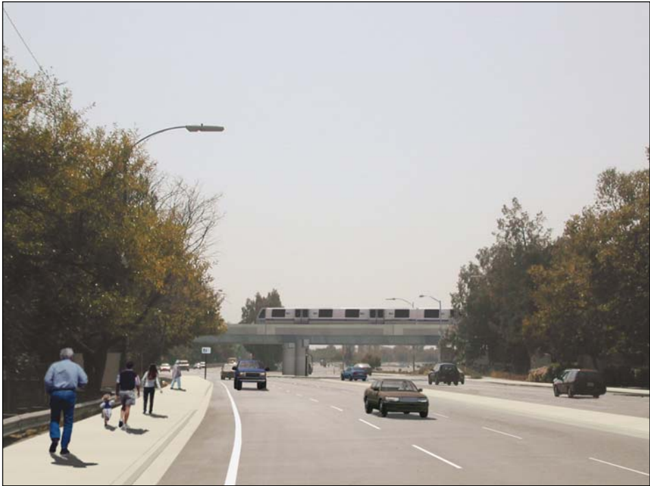
Figure 4.17-24: Berryessa Road Aerial Crossing (View to the southwest from Berryessa Road)
