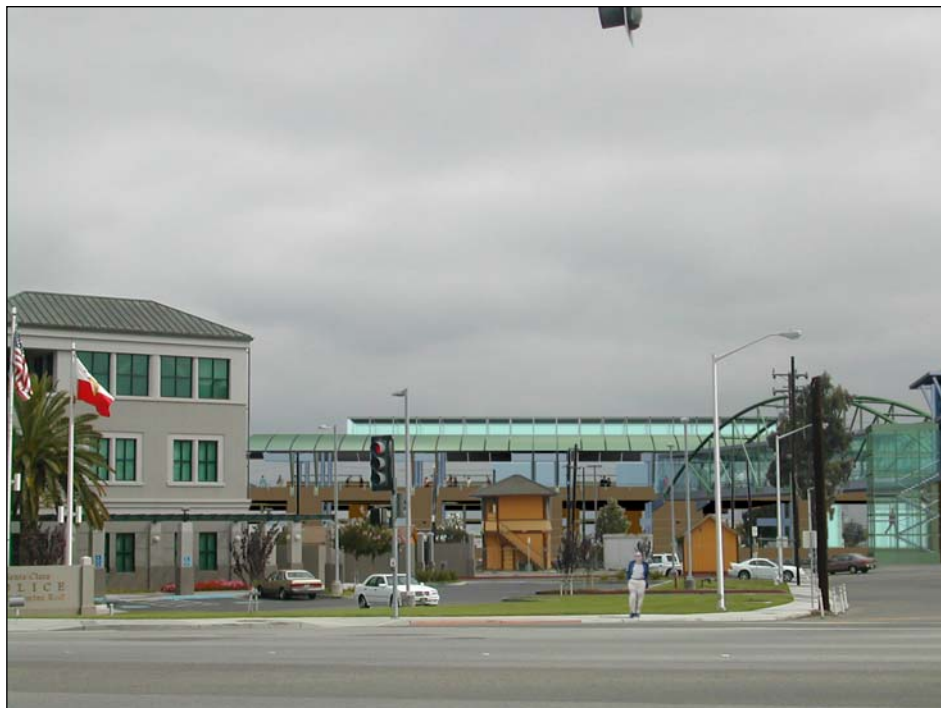
Figure 4.17-31: Santa Clara Station – Parking Structure North Option and Aerial Walkway South Option (View to the east from El Camino Real)
