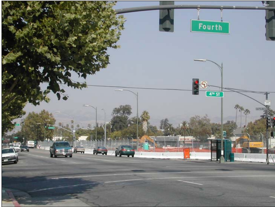
Figure 4.17-14: Civic Center/SJSU Station Location (View to the southeast from the corner of East Santa Clara Street and 4th Street)
