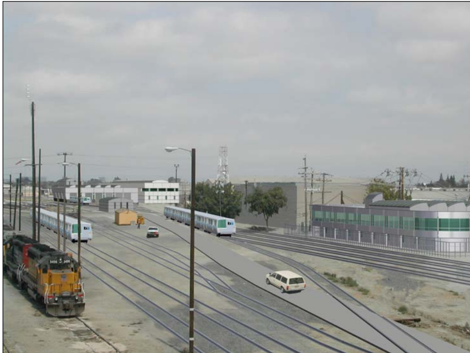
Figure 4.17-32: Maintenance Facility (View to the northwest from I-880)
