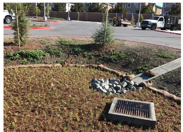
Bioswale at the Berryessa/North San Jose Transit Center.
