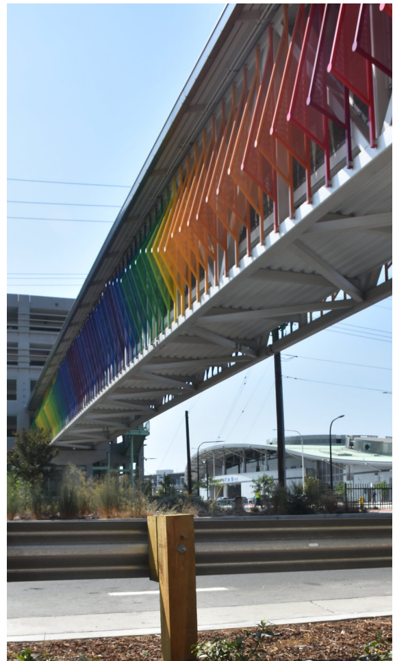
Montague Expressway Pedestrian Overcrossing
