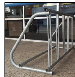
Wheel bender-type racks should be replaced
