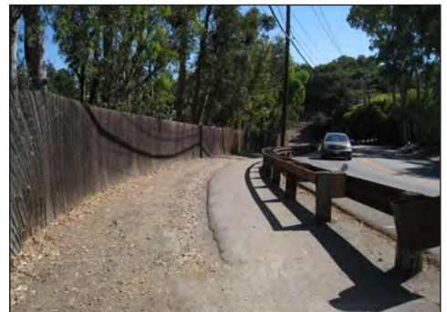
This roadside path in Los Altos Hills is separated from the roadway by a guard rail within the horizontal curve.
