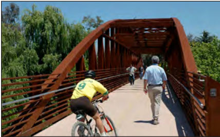
River Oaks Pedestrian/Bicycle Bridge over the Guadalupe River, opened May 2006, funded by 1996 Measure B.
