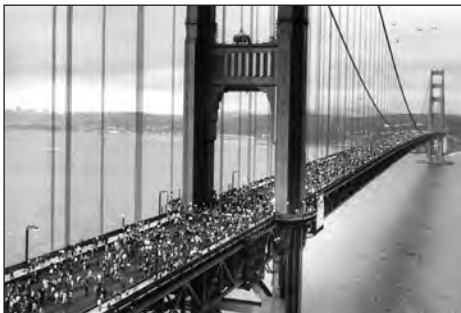
So many people crowded onto the Golden Gate Bridge during its 50th anniversary celebration in 1987 that it created the heaviest load the bridge had experienced to-date and its slight upward arch actually flattened under the weight; deflection is perfectly normal for any suspension bridge and this did not exceed the load capacity of the bridge.
