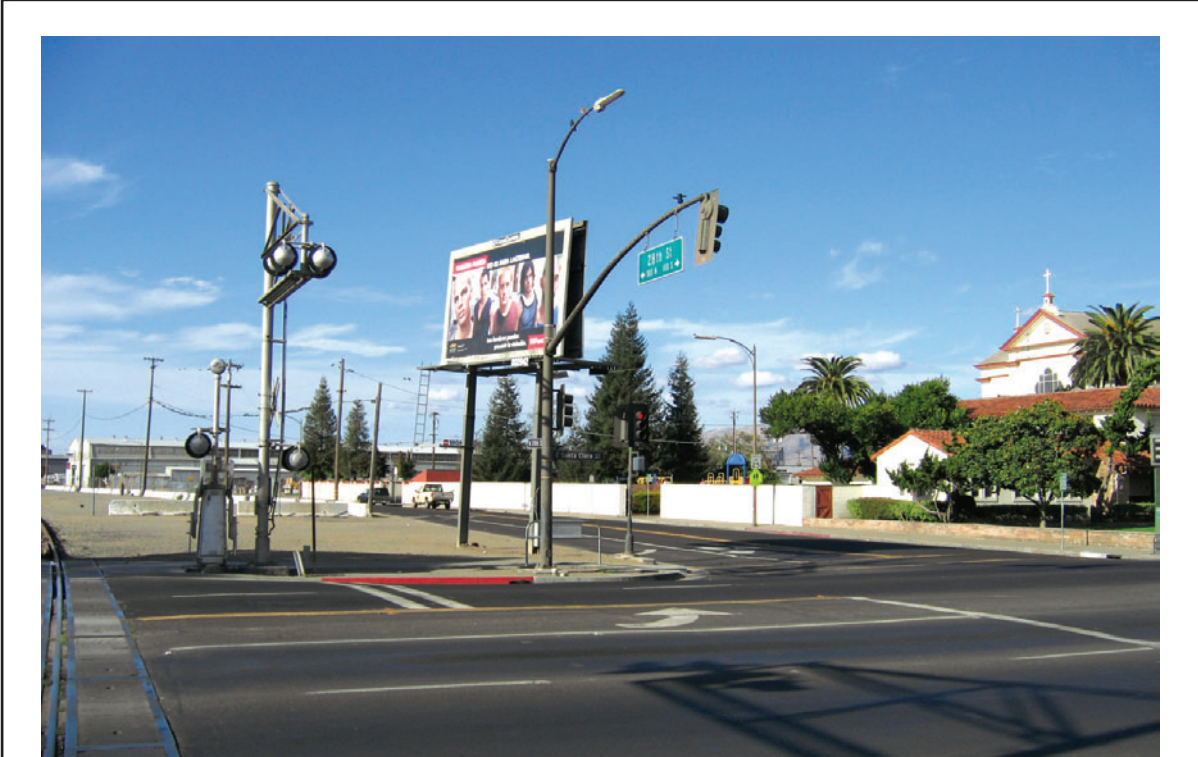
Existing View of Alum Rock Station and Parking Garage Location (view to the north from East Santa Clara Street)
