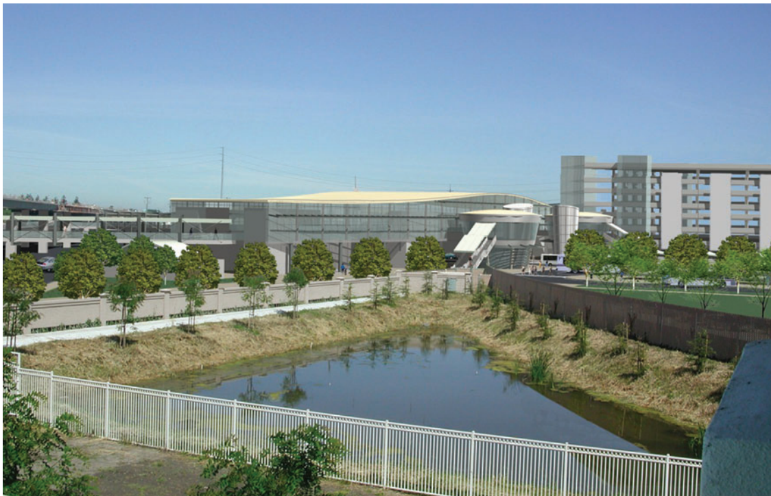
Visual Simulation of Milpitas Station (view to the northwest from “The Crossings at Montague” apartments)
