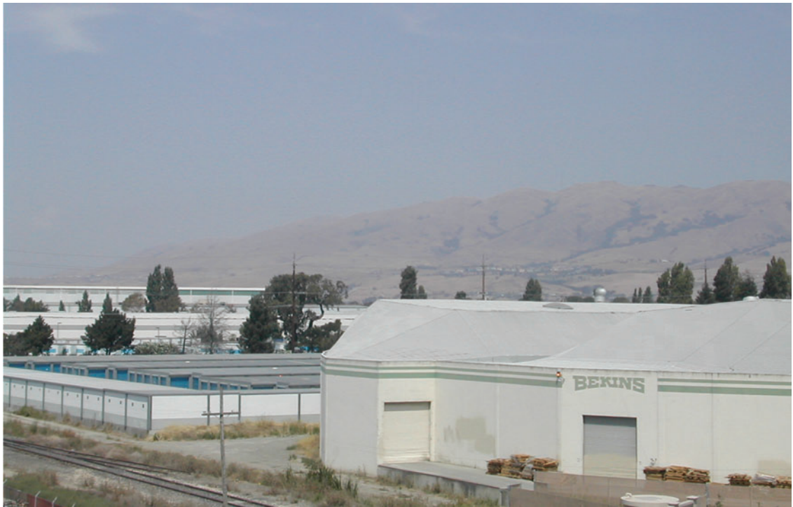
Existing View of Milpitas Station Location (view to the northeast from VTA Montague Light Rail Station)
