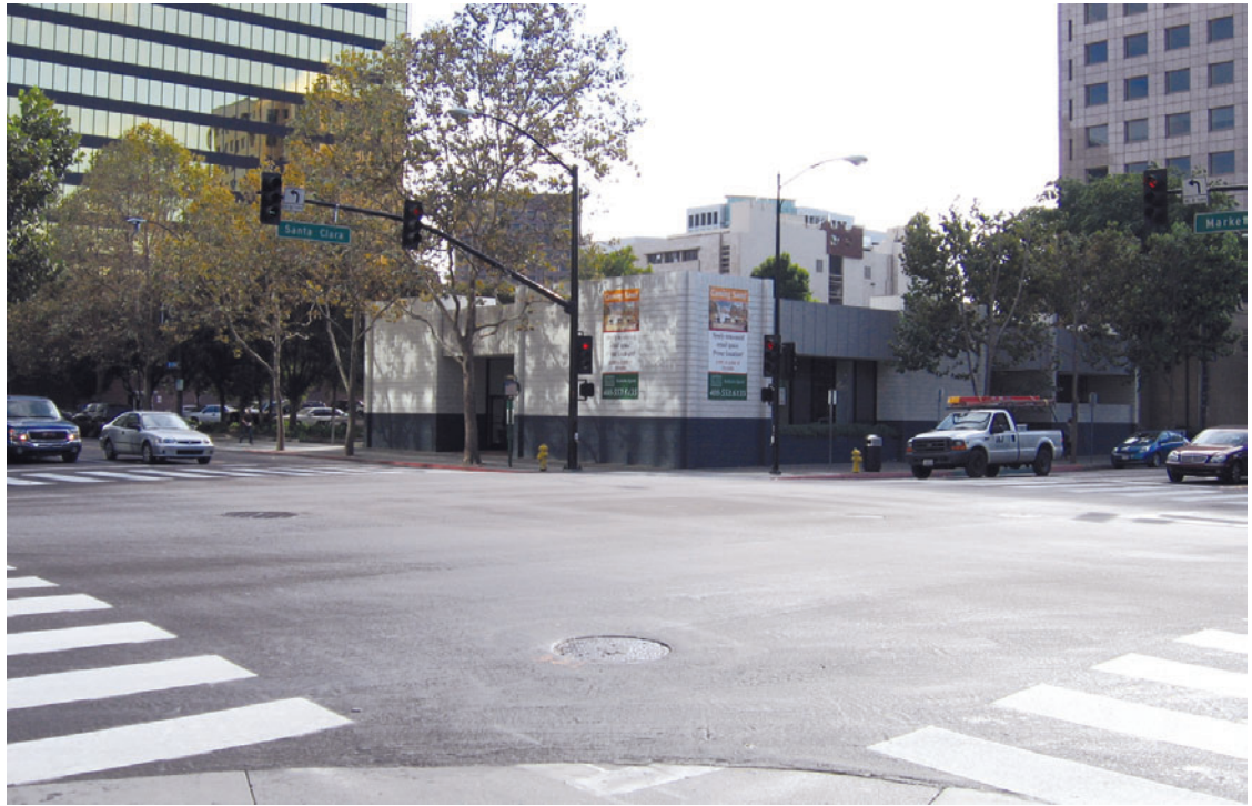
Existing View of Downtown San Jose Station Location (view looking southwest from northeast corner of Market Street and Santa Clara Street)
