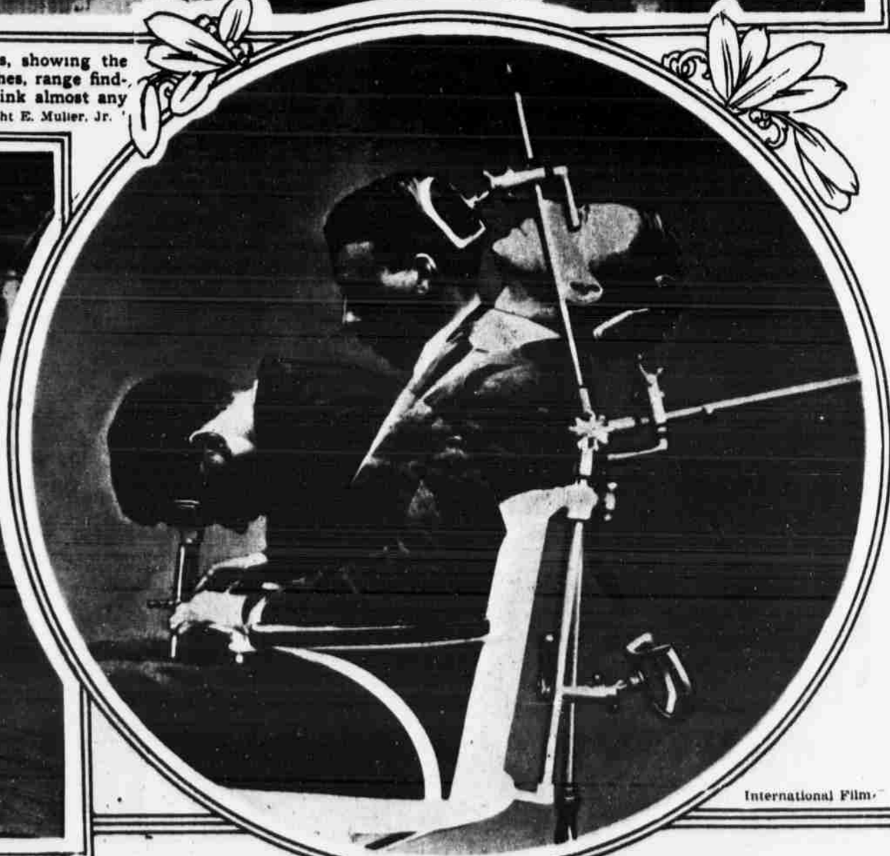
Composite photograph showing three positions in which aviation candidates are examined for the vital "sense of balance." The chair and aspirant are revolved rapidly, and any sign of vertigo bars him.
