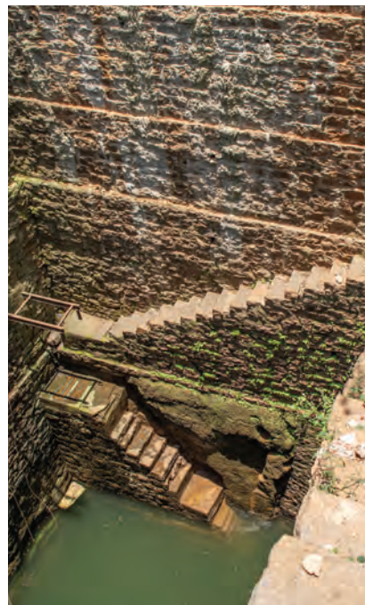
Rejuvenated stepwells provide better groundwater access for communities.
