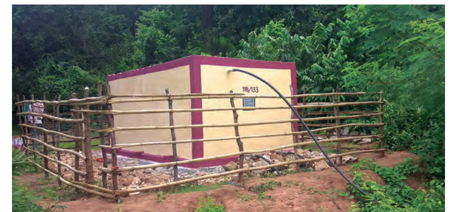
The water supply system ensures proper filtration of water captured at source and also allows for storage.
