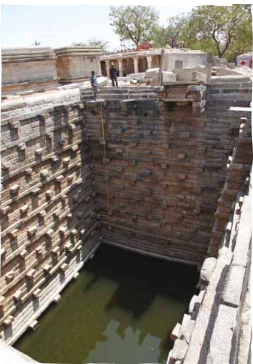
Open well at Lakshmeshwara
