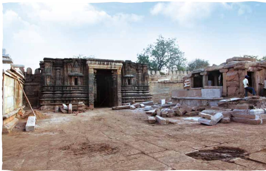
Restoration work underway at Lakshmeshwara
