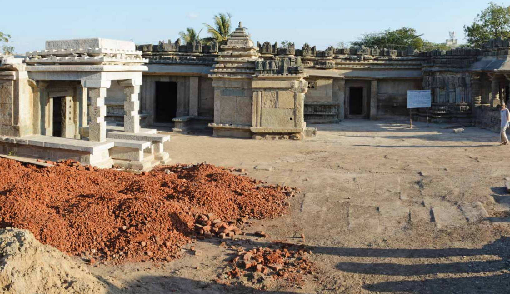
Restoration work underway at Lakshmeshwara
