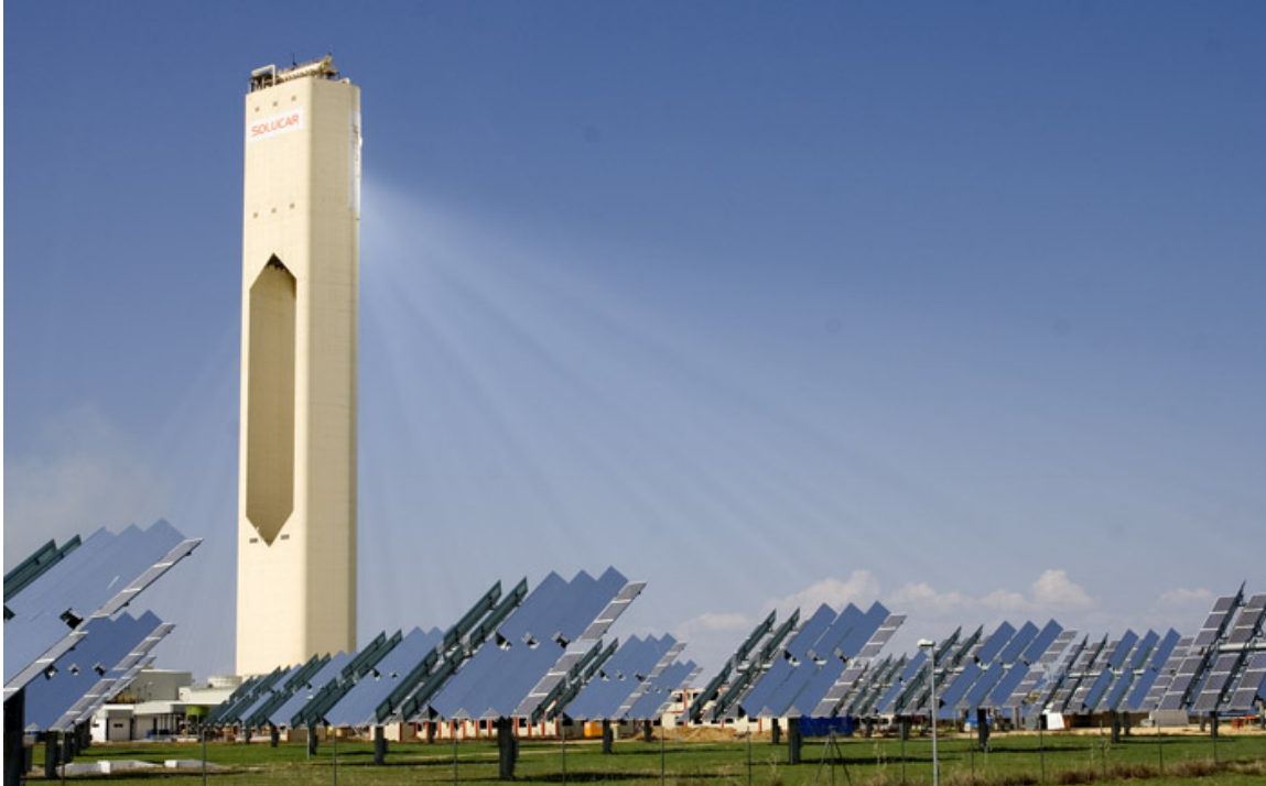
Power Tower Example: the PS10 system located in Spain (Image courtesy of afloresm , Wikimedia Commons, 2007)
