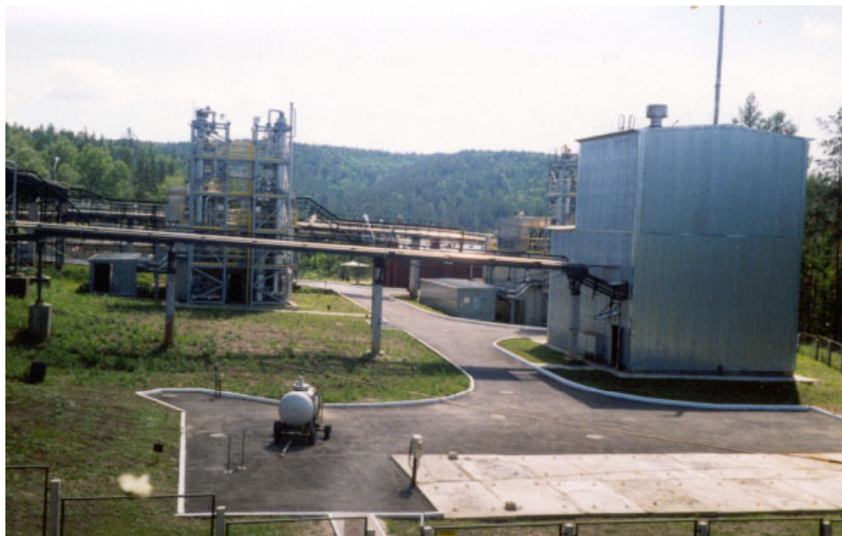
Ground View of the Heptyl Fuel Disposition System
