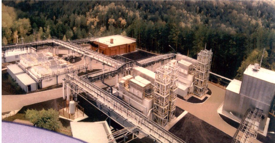
Aerial view of the Heptyl Disposition Systems and Infrastructure
