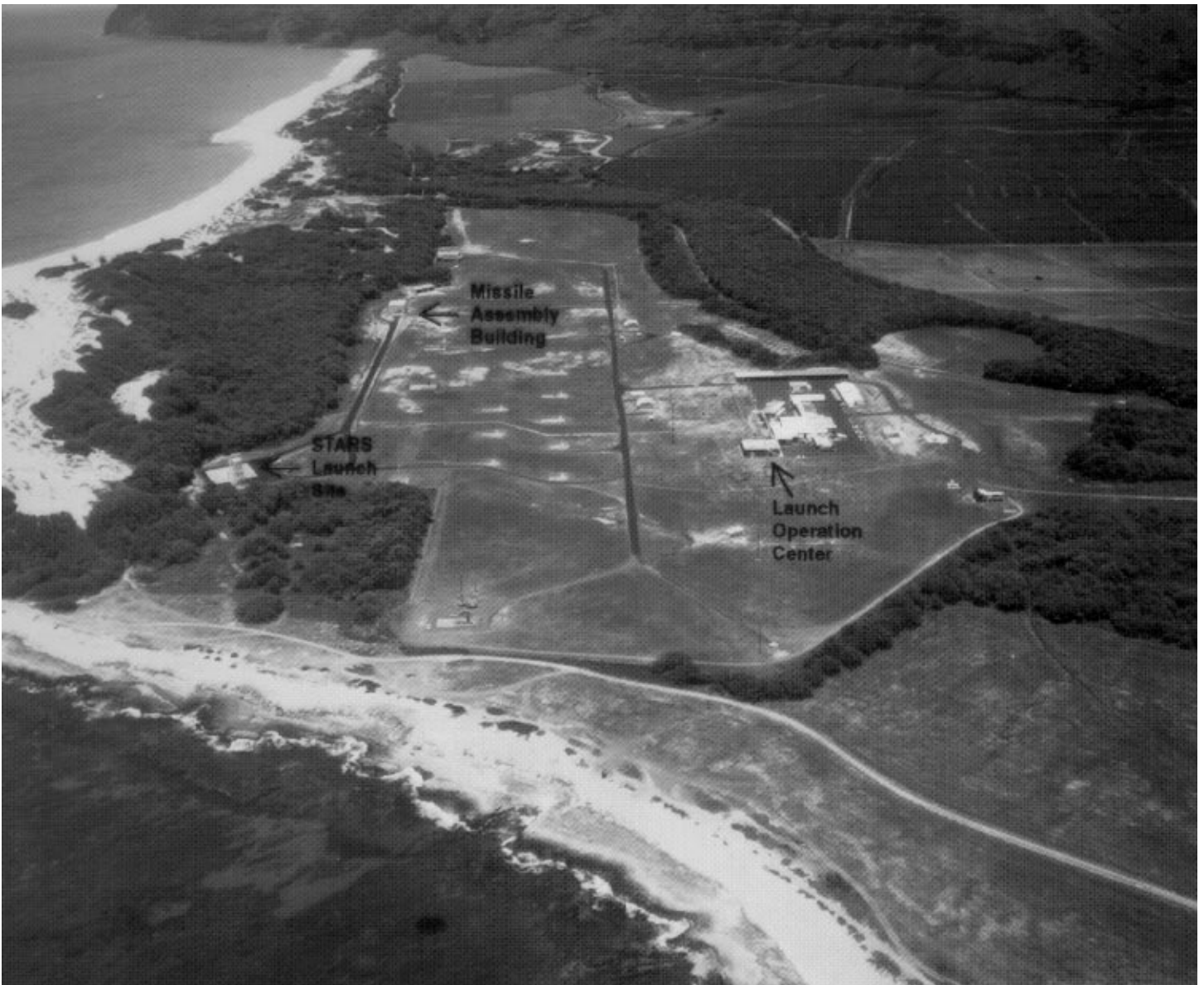
Figure I.3: Aerial View of Kauai Test Facility
