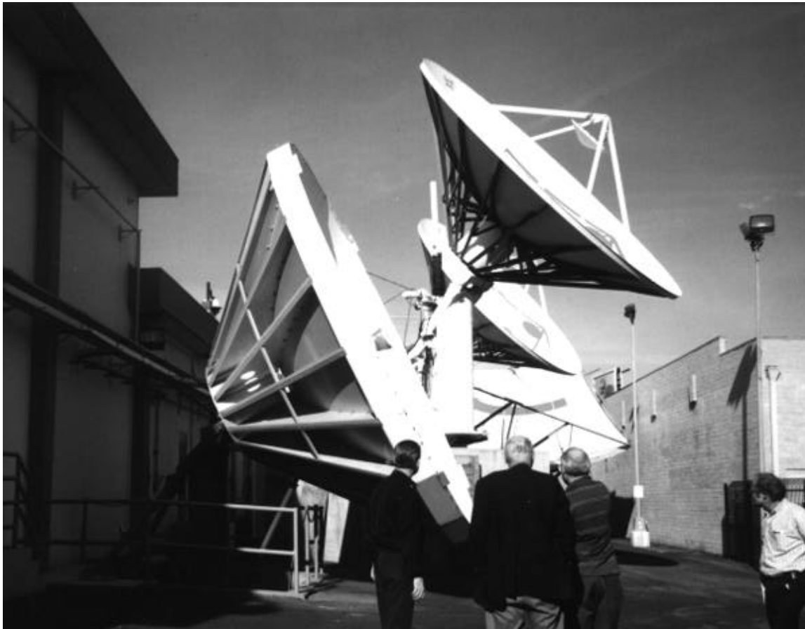
Figure 5. Existing emitting antenna (foreground) and receiving antennas at Sun Valley facility.
