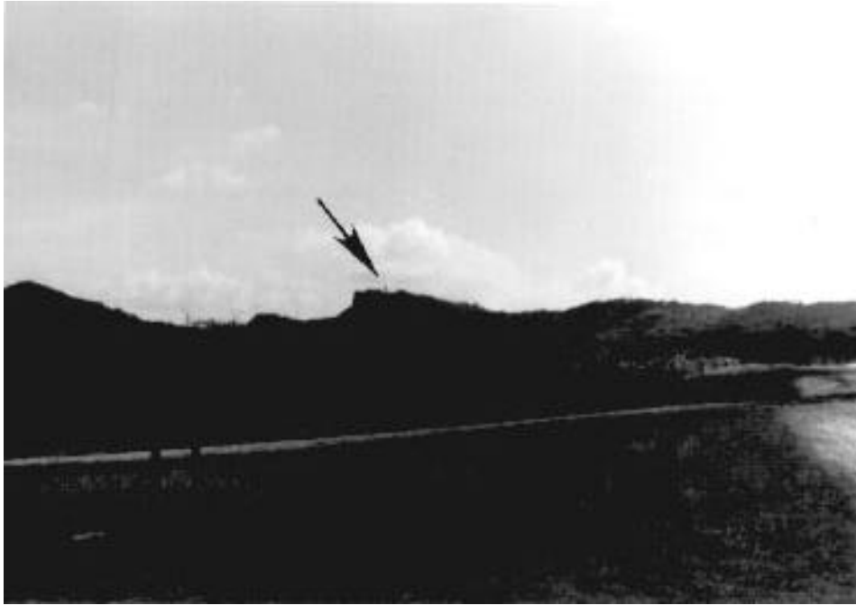
D.1 Looking South from Grotto Junction Radar Facility in Center of Photo
