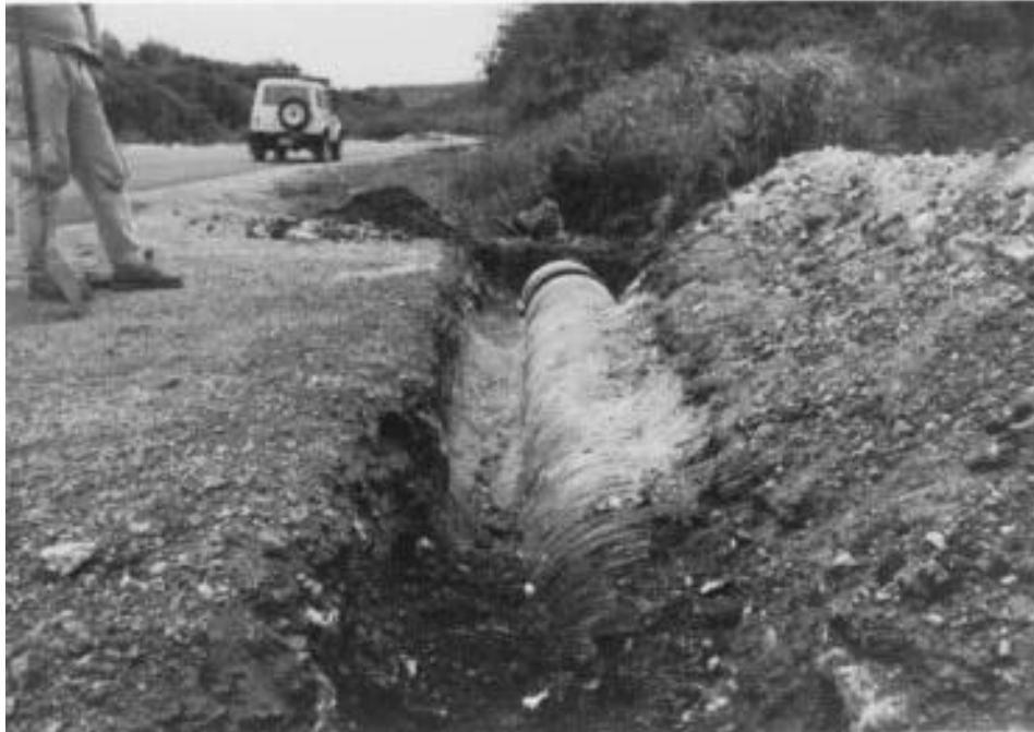
D.17 Looking East at Cleanout of Existing Roadside Culvert
