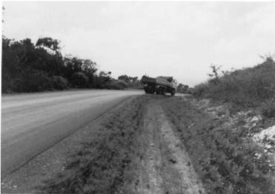
D.8 Looking West at Grass-lined Ditch near Junction of Forest Roads 500 and 530
