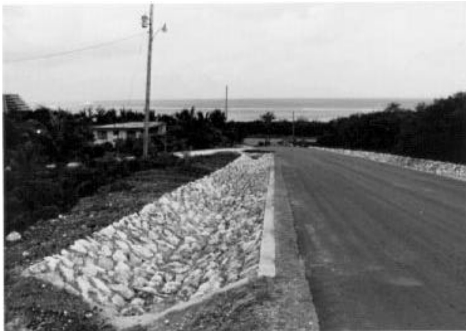
D.18 Looking West into Riprap-lined Ditch to Culvert V Inlet
