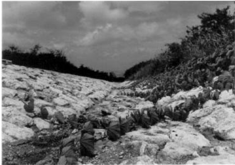
D.16 Looking West into Riprap-lined Ditch Downgradient of Culvert IV
