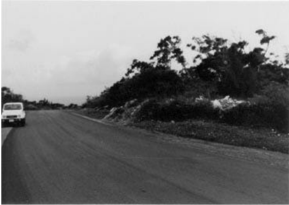
D.21 Looking West toward Blockage of Forest Road 540
