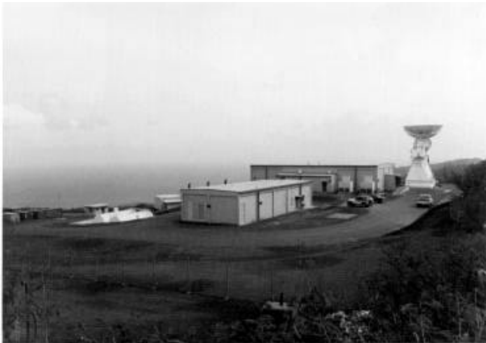
D.29 Looking Northwest toward Radar Site Post-construction
