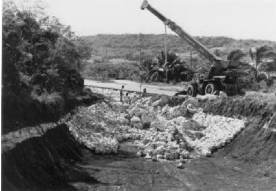
D.19 Looking Southeast into Stilling Basin Riprap Placement
