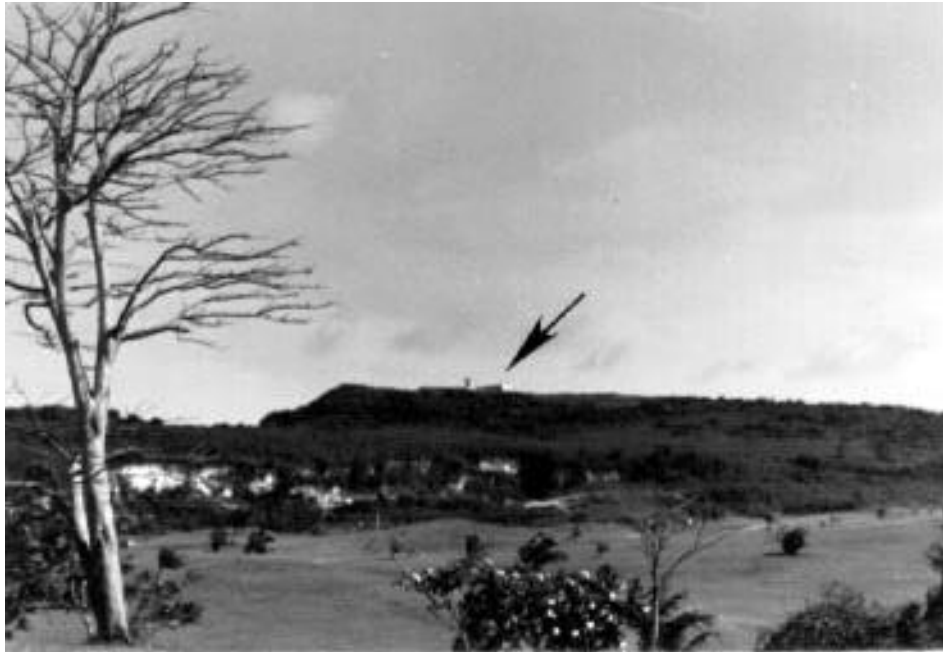
D.4 Looking Southeast from Golf Course Radar Facility atop Hill at Center of Photo
