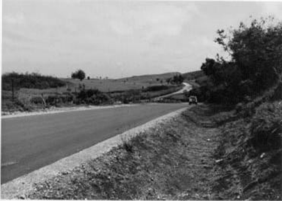
D.13 Looking North from Grass-lined Ditch Upgradient of Culvert III
