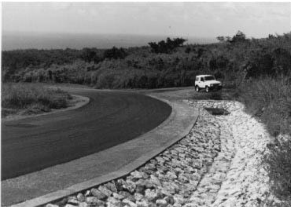
D.12 Looking Northwest at Riprap-lined Ditch and Culvert I Inlet
