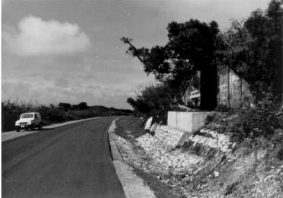
D.9 Looking North toward Erosion Protection at World War II Bunker
