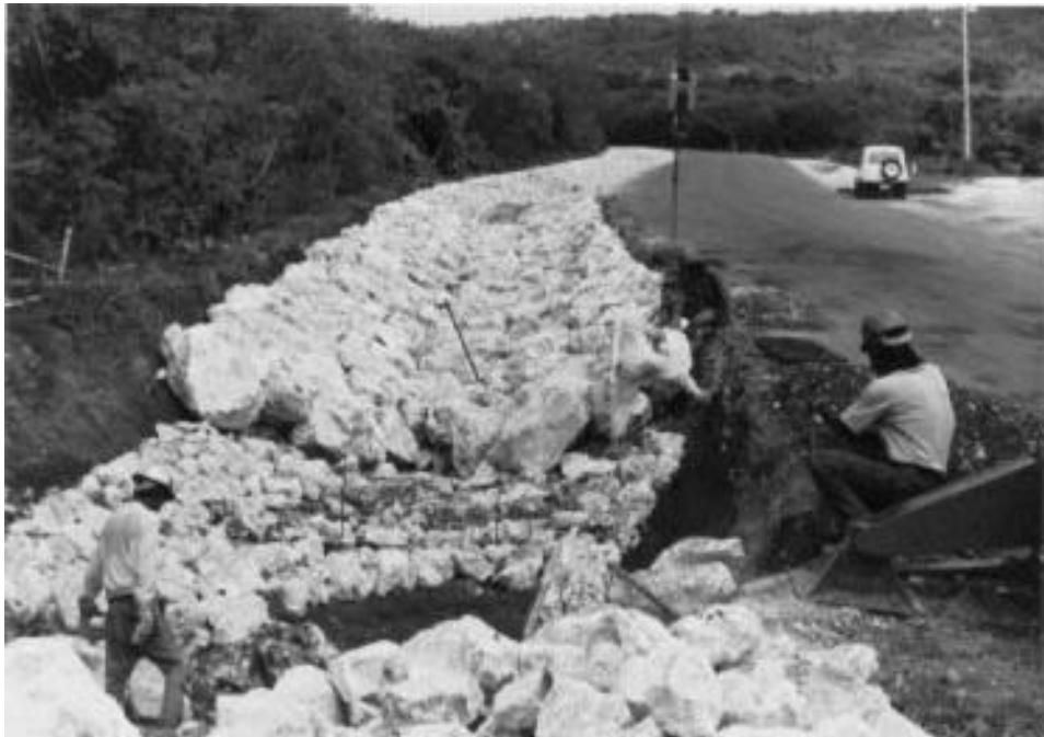
D.20 Looking East into Stilling Basin Riprap Placement
