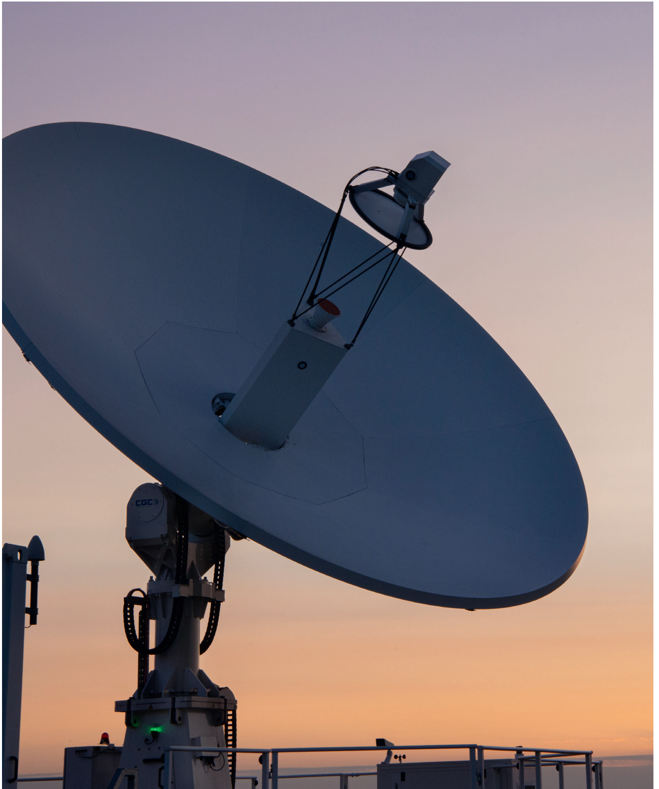
Dstl Hermes Ground Station, Portsmouth West, Hampshire 20
