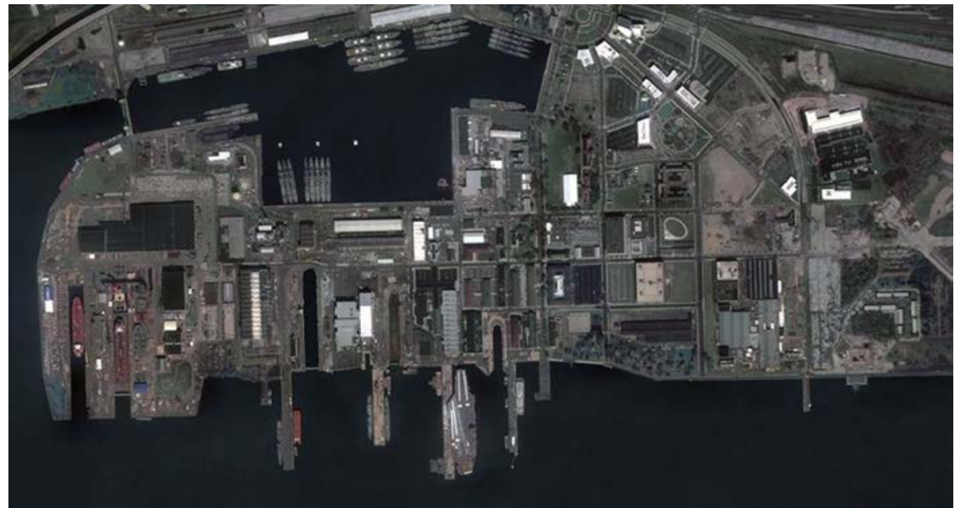
Naval Inactive Ship Maintenance Facility in Philadelphia, PA
