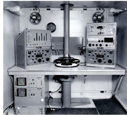
Figure 8. Interior of a GRAB hut
