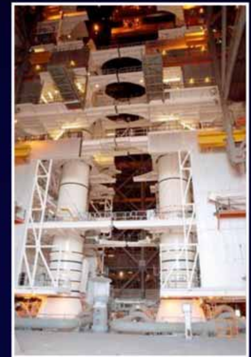
SRB Stacking Complete
