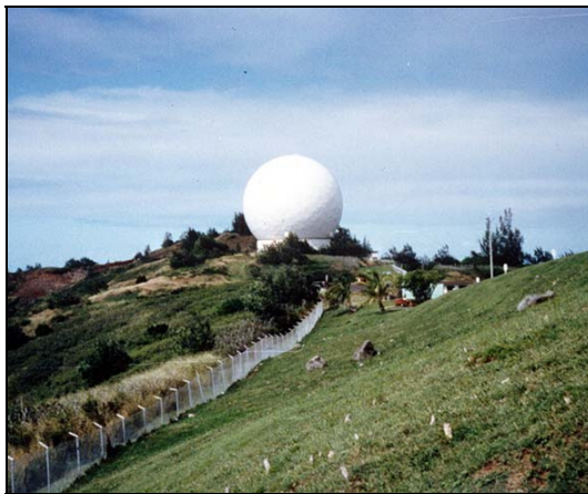
Fig. 21-10. Kaena Point Tracking Radar
