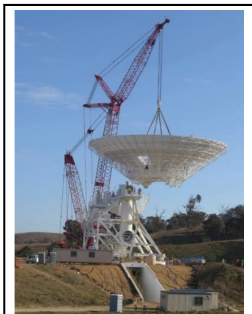
The main reflector lift for Deep Space Station (DSS)-36 at Canberra Deep Space Communications Complex, readies NASA for deep space communications operations for the next decade.
