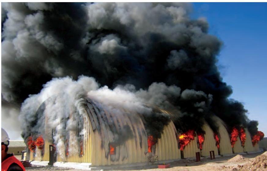
A fire at a non-code-compliant ANA classroom destroyed the structure in 30 minutes. See Special Project 14-77-SP. (USACE photo)
