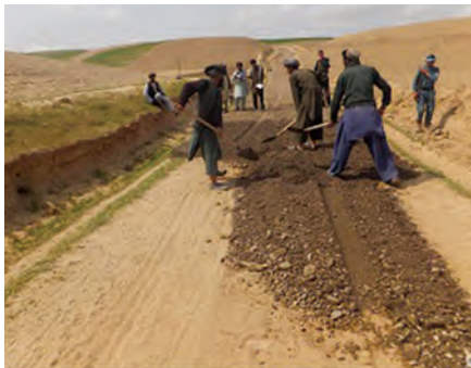
SIKA West road-rehabilitation project in Muqur District, Badghis Province. (USAID photo)
