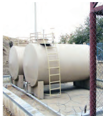
Despite water and sewage system problems, as well as electrical concerns, the Sheberghan school is already in use by Afghans. (SIGAR photo)
