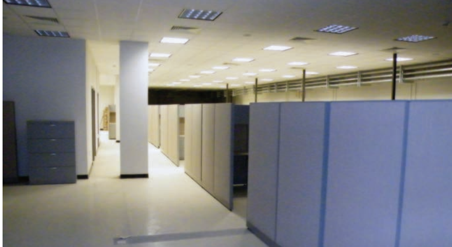
Cavernous and unneeded by the U.S. military, a $34 million command-and-control complex with an acre and a half of floor space sits idle in Helmand Province, with no current plans for alternative use. (SIGAR photo)
