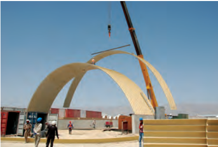
Workers construct a K-span building at Bagram Airfield. (U.S. Army photo)
