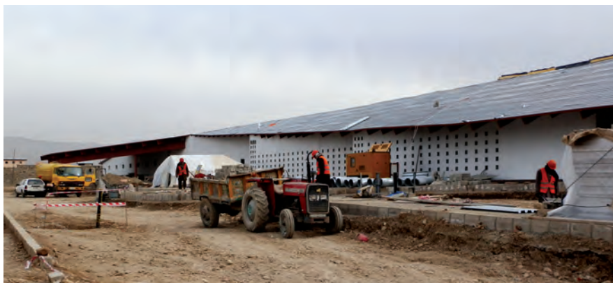
Gardez hospital under construction. (SIGAR photo)
