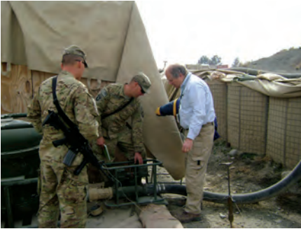
Special IG Sopko examines fuel pumping at FOB Salerno. (SIGAR photo)
