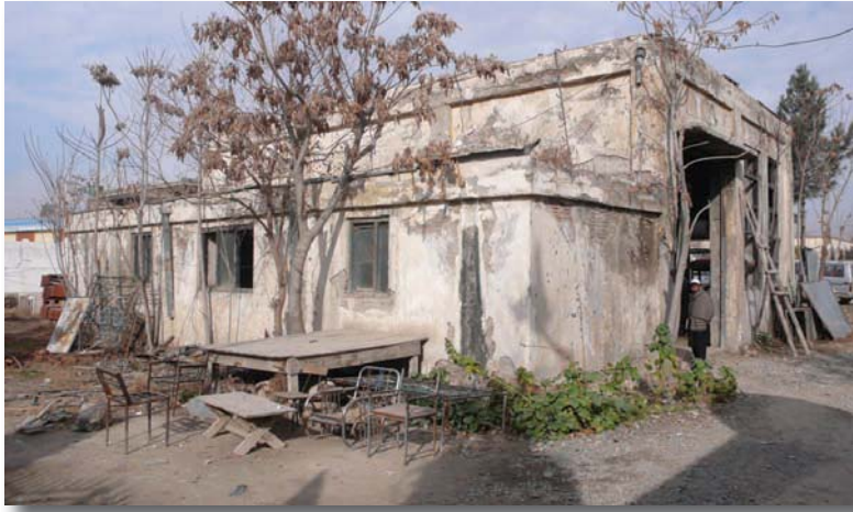
Original condition of the Khowst power plant in Jan 2008
