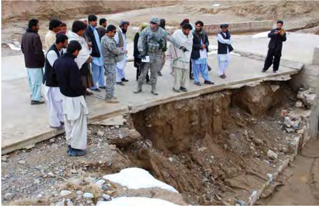
U.S. Air Force Tech. Sgt. Latha Caillouette, a PRT Zabul structures engineer, shows contractors erosion control repairs that are needed at a bridge in Shah Joy District, Zabul Province, on March 4, 2011. (U.S. Air Force photo by 1st Lt. Brian Wagner)
