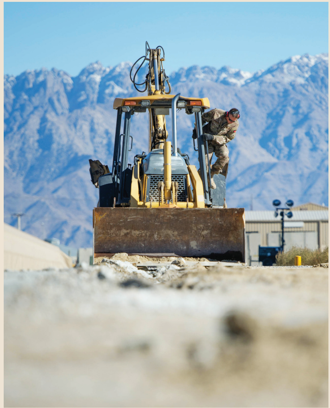
A member of a U.S. civil-engineering squadron checks his backhoe at Bagram Airfield. (USAF photo by Tech. Sgt. Robert Cloys)
