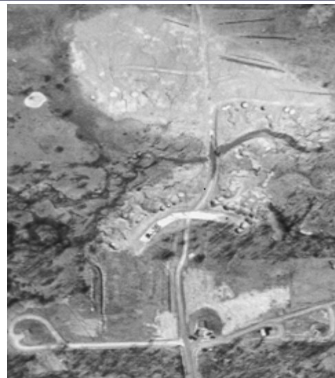
Aerial Photo of the Demolition Area #2.
