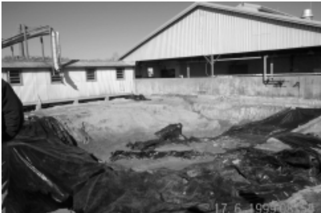
View of Excavated Soil Inside of Production Load Line
