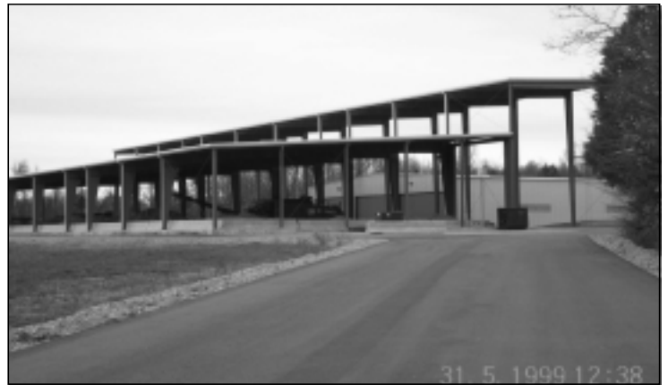
Exterior View of Composting Facility
