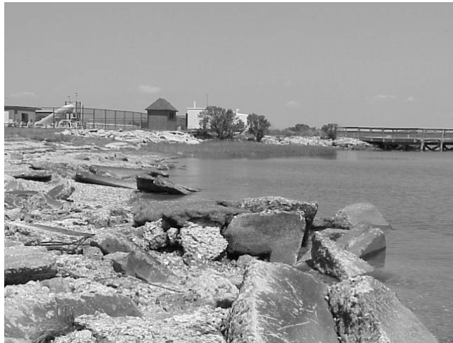
Figure 2-1. LTA Pool and Sewage Pump Station.
