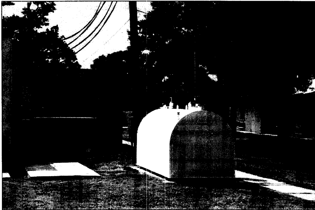
July 17, 2000. Heat. Pump east of Building 142 , adjacent to Parcel E1. Photo taken facing west.
