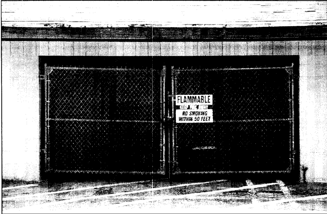
July 17, 2000. Inside view of lawn mower storage building. Building located northeast of Building 138 , adjacent to Parcel E1. Photo taken facing west.
