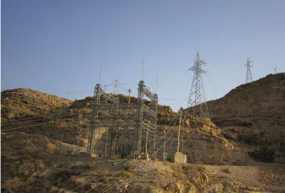
Insurgent attacks are also focused on non-military targets, including power transmission lines. (USACE photo)
