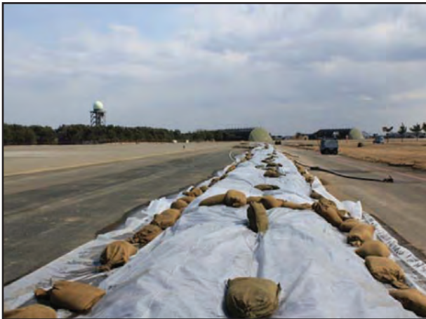
Figure 1-7. If radiological levels are remonitored and unable to be brought under published threshold levels, the aircraft, vehicle, or equipment will be transported to the hot cargo pad (above) for isotope identification, further radiological analysis, and gross decontamination.
