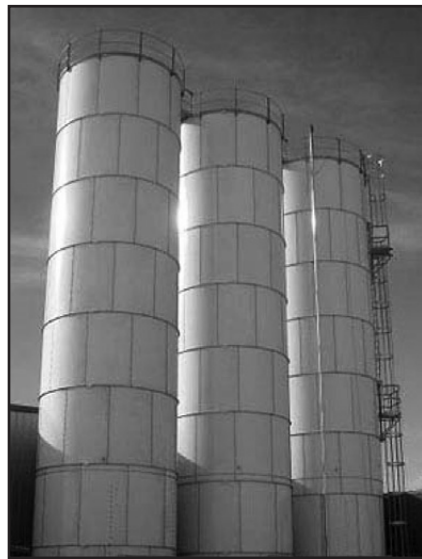
Figure 5-4. Standpipe towers. These are probably chemical process standpipes.
