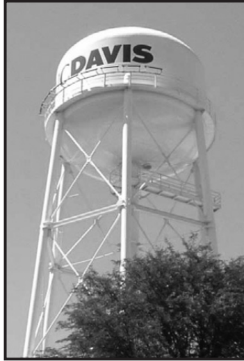
Figure 5-3. Common water tower
