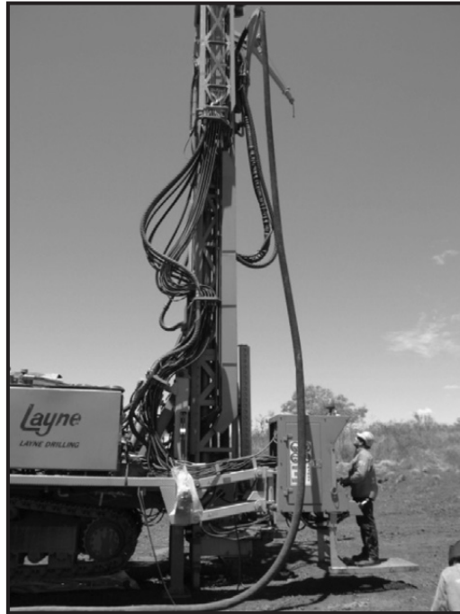
Figure 5-2. Well-drilling rigs can be tracked or wheeled.
