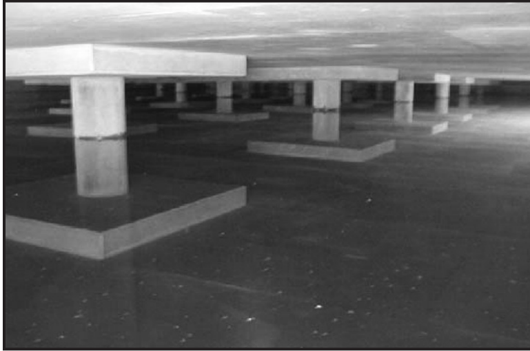
Figure 5-5. Underground storage reservoir (wet well)
