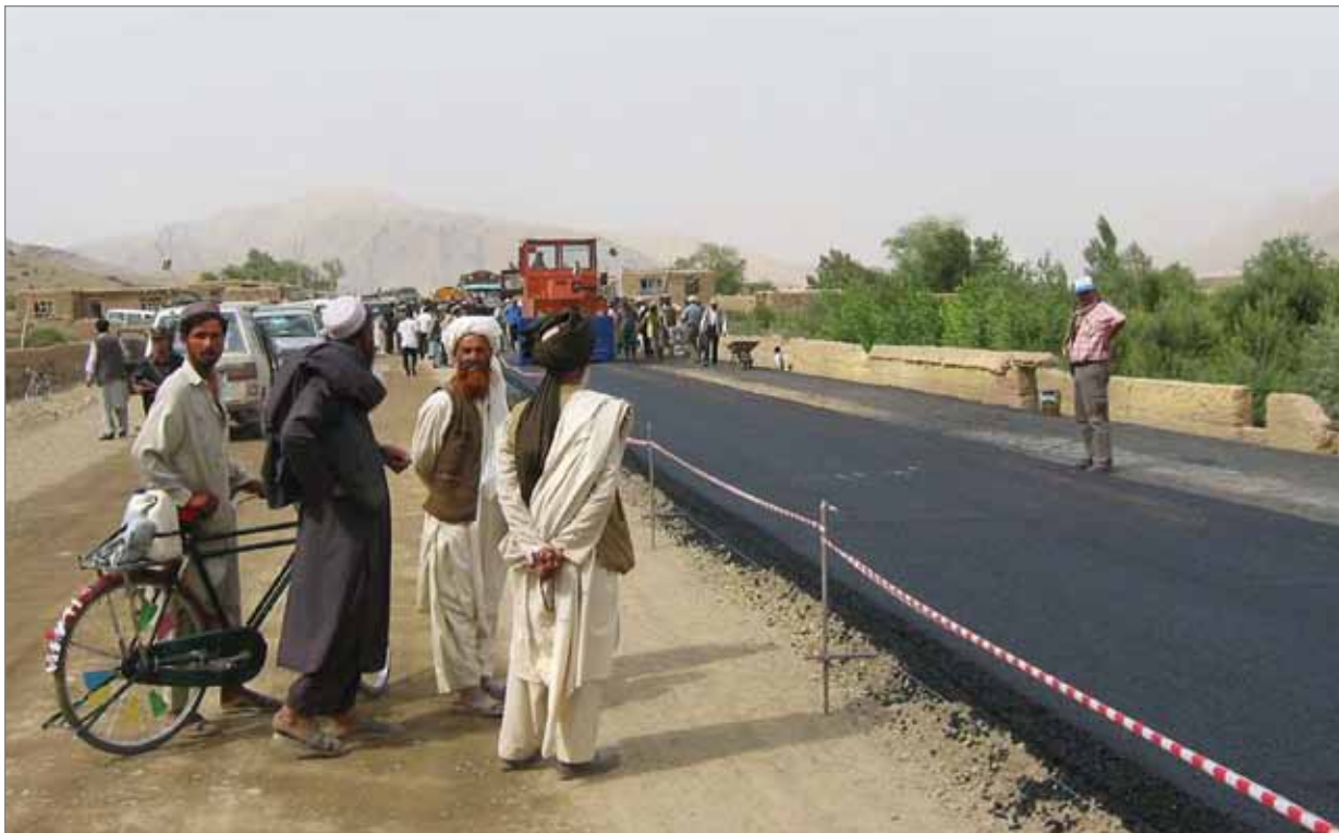
Kabul-to-Kandahar road construction, 2003. (USAID photo)
