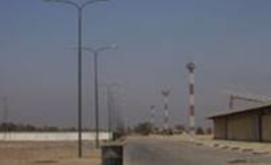
Lights and Power Poles
