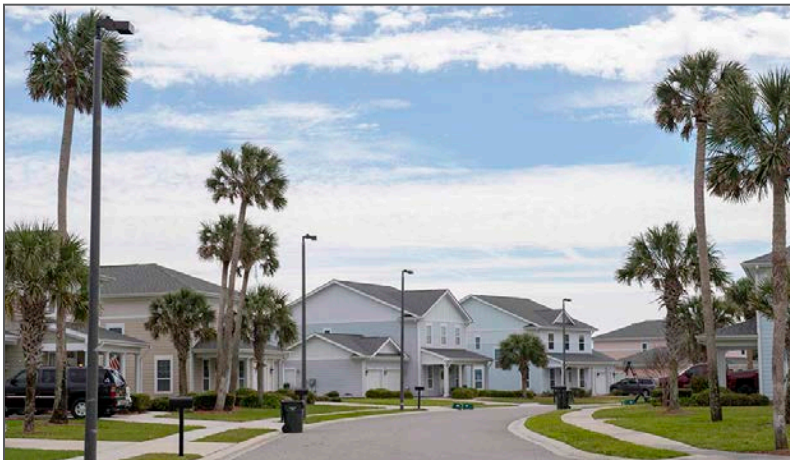
Homes at Bennett Shores East, an on-base military housing community at Naval Station Mayport, Florida, March 18, 2019.
