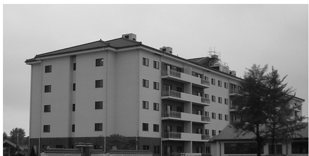
Figure 1 -- New family housing unit at Camp Humphreys
