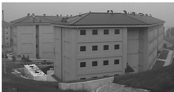
Figure 2 -- New dormitory at Osan Air Base
