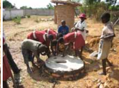
The pit is lined with bricks and the slab fitted. Space between bricks and pit wall backfilled with soil and rammed hard.
