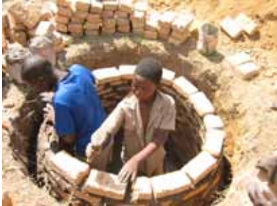
The pit is lined with bricks and the slab fitted. Space between bricks and pit wall backfilled with soil and rammed hard.
