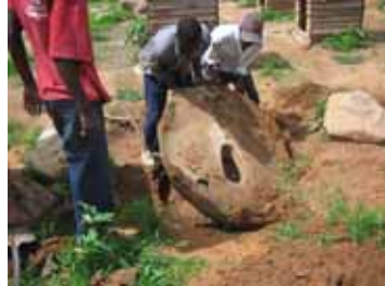
A series of Arborloo's at a school site. Slab being removed from full pit.
