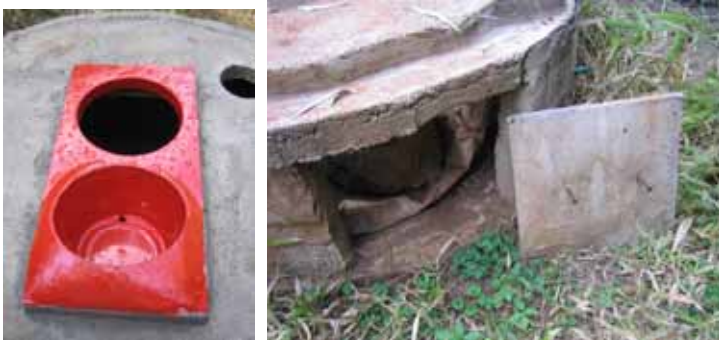
Urine diverting squat plate and vault door.
