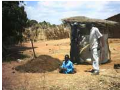
Excavating pit compost in Mozambique and Malawi
