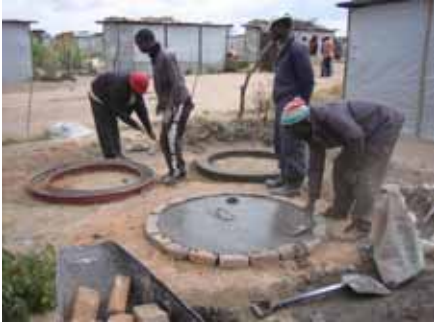
Two ring beams and a single slab are cast for the alternating pit system
