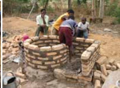
Foundations laid outside the slab and walls built on top.
