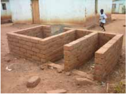
Double vault system being built in Lilongwe, Malawi. In this case the toilet is coupled with a washroom. Programme by CCODE Malawi.
