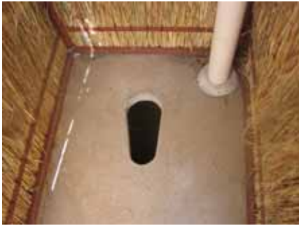
Left: Round slab fitted with rectangular grass walled steel frame structure and PVC pipe. Right: brick structure fitted with cement pipe.
