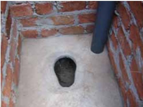
The interior can be fitted with a standard squat hole or upgraded with a pedestal. There are many ways of making a home made pedestal using cement, a bucket and a seat.
