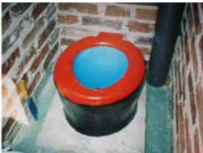
Pedestal made from concrete and a plastic bucket inside brick structure with PVC pipe. On right urine diverting pedestal fitted over pit toilet.
