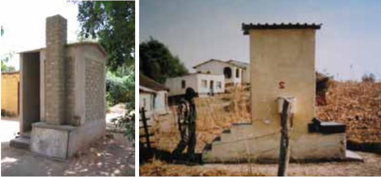
Single vault urine diverting toilet built by Mvuramanzi Trust, Zimbabwe. Early single vault urine diverting toilet built in South Africa. South Africa has built the largest number of urine diverting systems in Africa.
