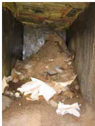
The vault door is opened to reveal the vault contents. These require extra processing before they can be used. CCODE Malawi.
