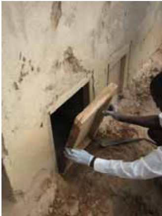
The vault door is opened to reveal the vault contents. These require extra processing before they can be used. CCODE Malawi.
