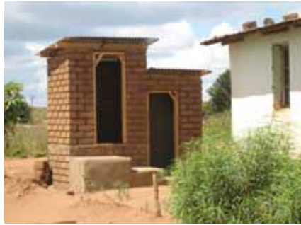
Double vault system being built in Lilongwe, Malawi. In this case the toilet is coupled with a washroom. Programme by CCODE Malawi.
