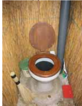
The interior can be fitted with a standard squat hole or upgraded with a pedestal. There are many ways of making a home made pedestal using cement, a bucket and a seat.
