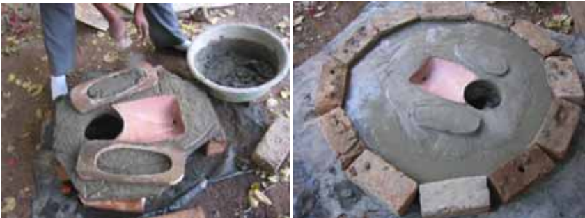
Urine diverting squat plate and vault door.
