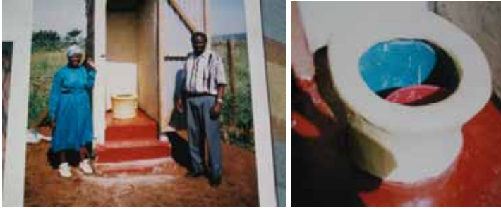
Home made toilet and urine diverting pedestal in Kenya
