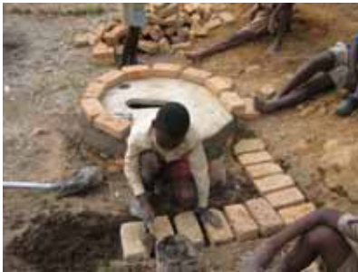
Foundations laid outside the slab and walls built on top.
