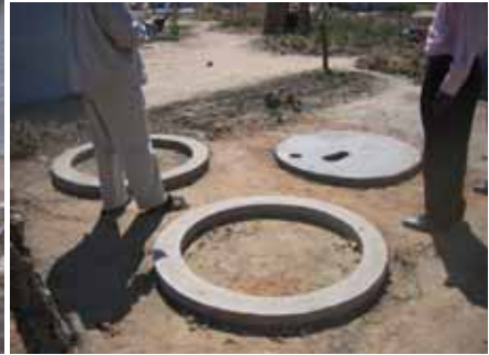
Two ring beams and a single slab are cast for the alternating pit system
