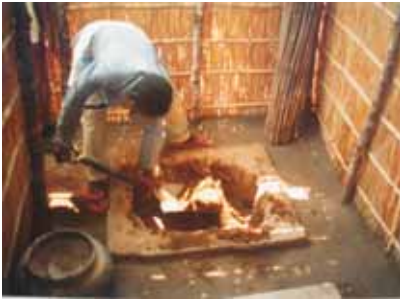
Excavating pit compost in Mozambique and Malawi
