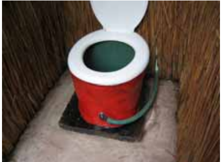
Pedestal made from concrete and a plastic bucket inside brick structure with PVC pipe. On right urine diverting pedestal fitted over pit toilet.
