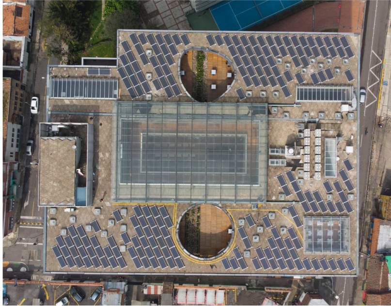
Figure 1: PV system at Universidad de los Andes. Taken from [14].
