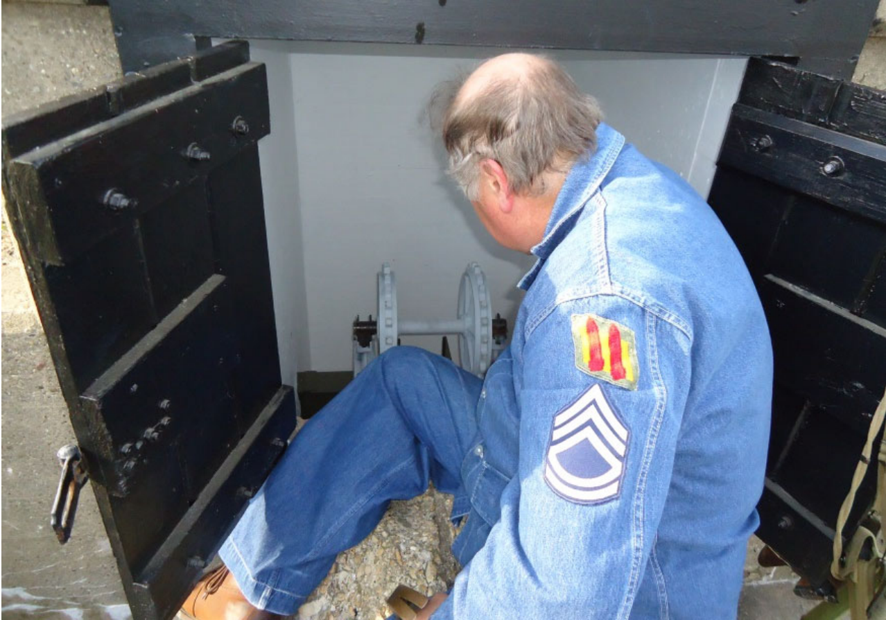
Below the upper sprocket and shaft is in place on the two trunnion mounts.
