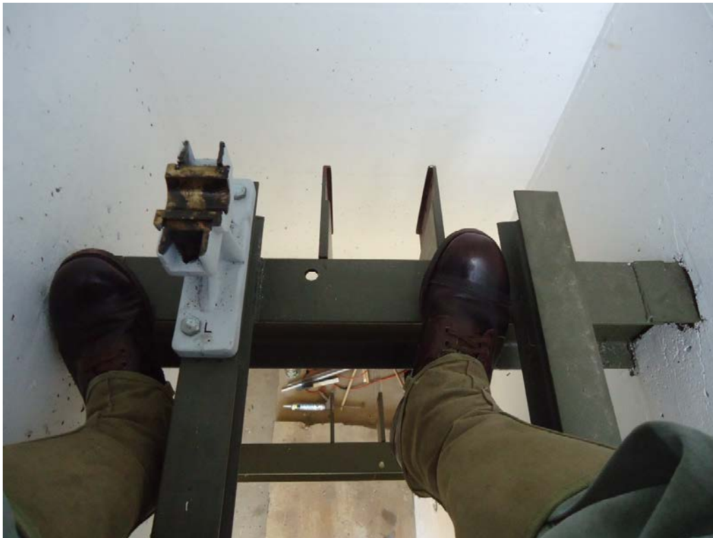
The left trunnion base is shown with a bolt in place.
