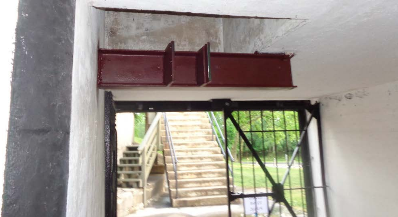
The lower 7-inch I-Beam as seen from the entrance to the magazine.
