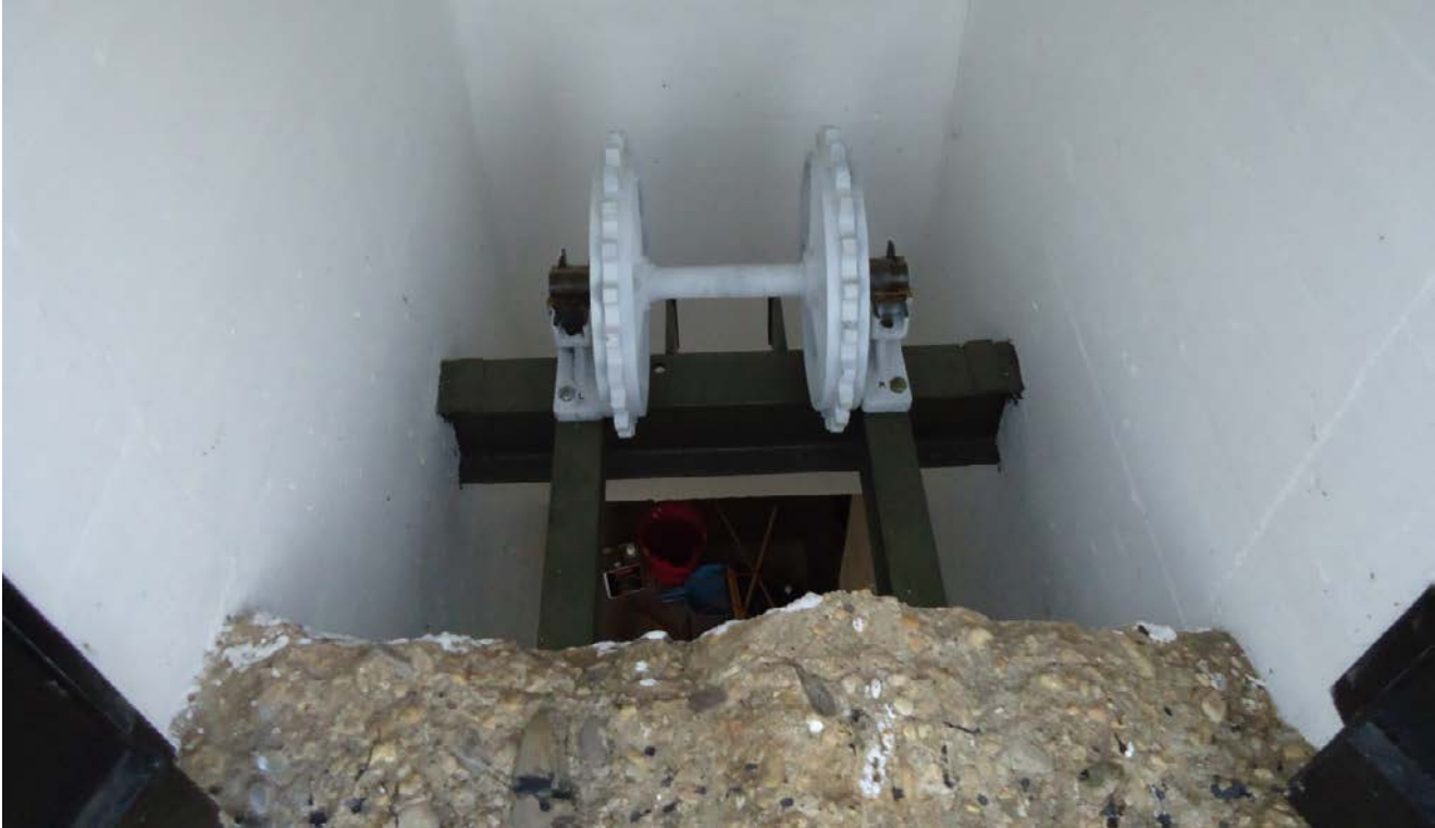
Below the upper sprocket and shaft is in place on the two trunnion mounts.
