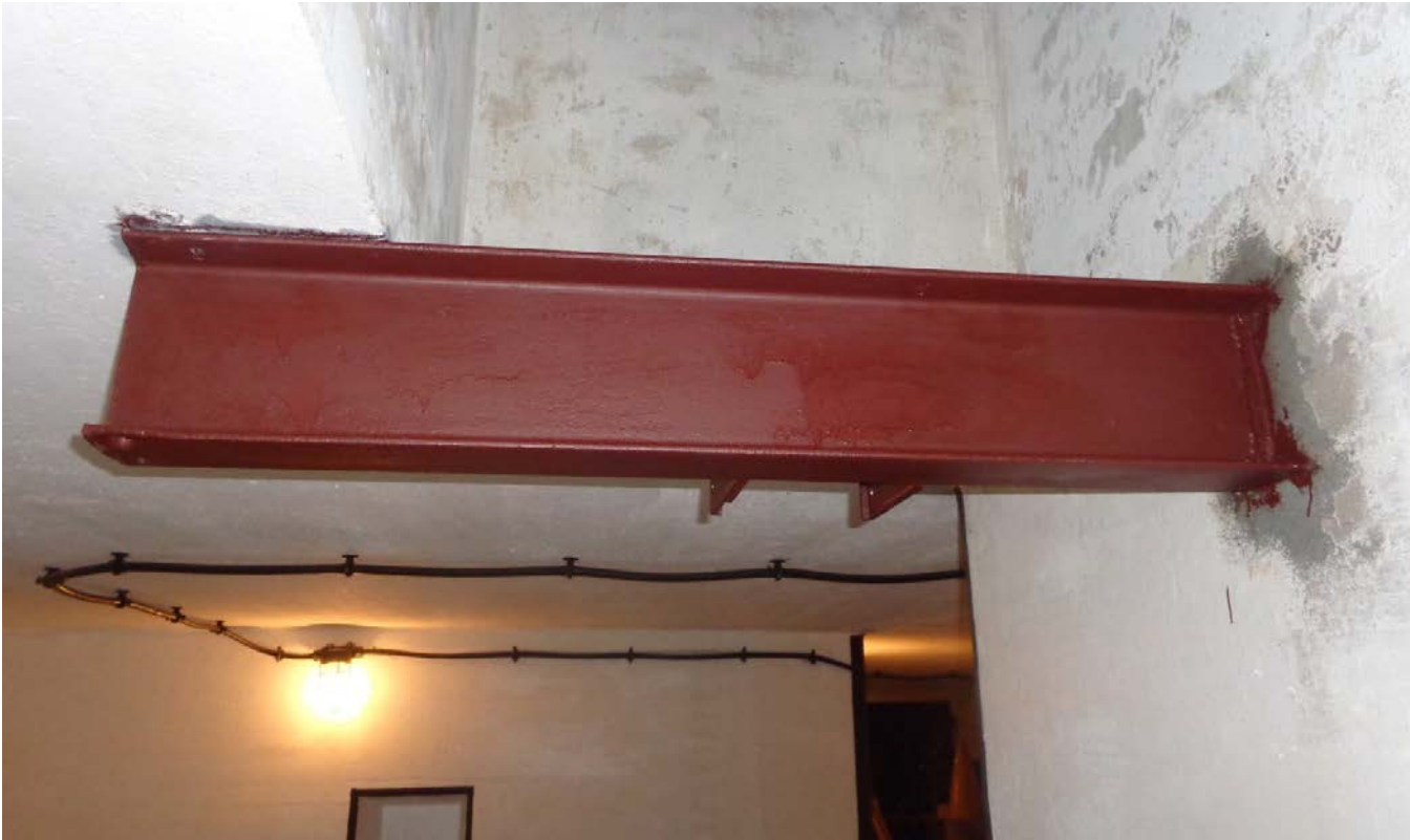
The lower 7-inch I-Beam as seen from the entrance to the magazine.
