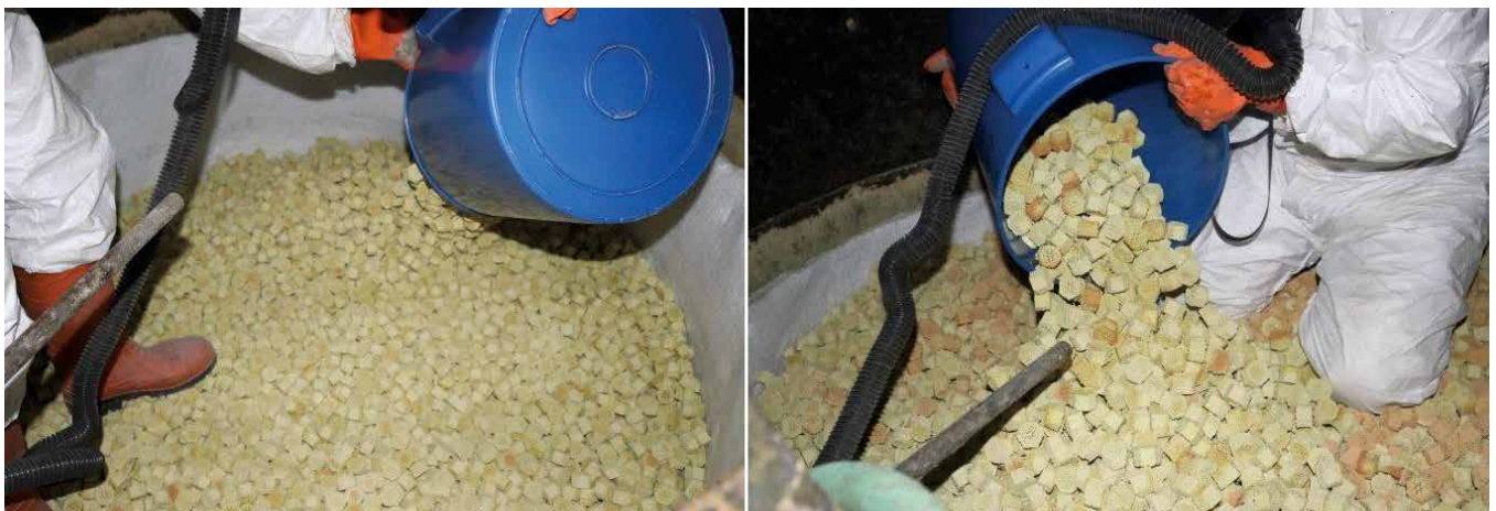
Fig. 3: Filling of the O4-115 X3D™ catalyst into bed 3 of the converter at the BASF reference plant.
