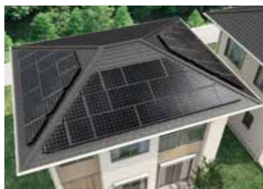
Solar power generation systems
