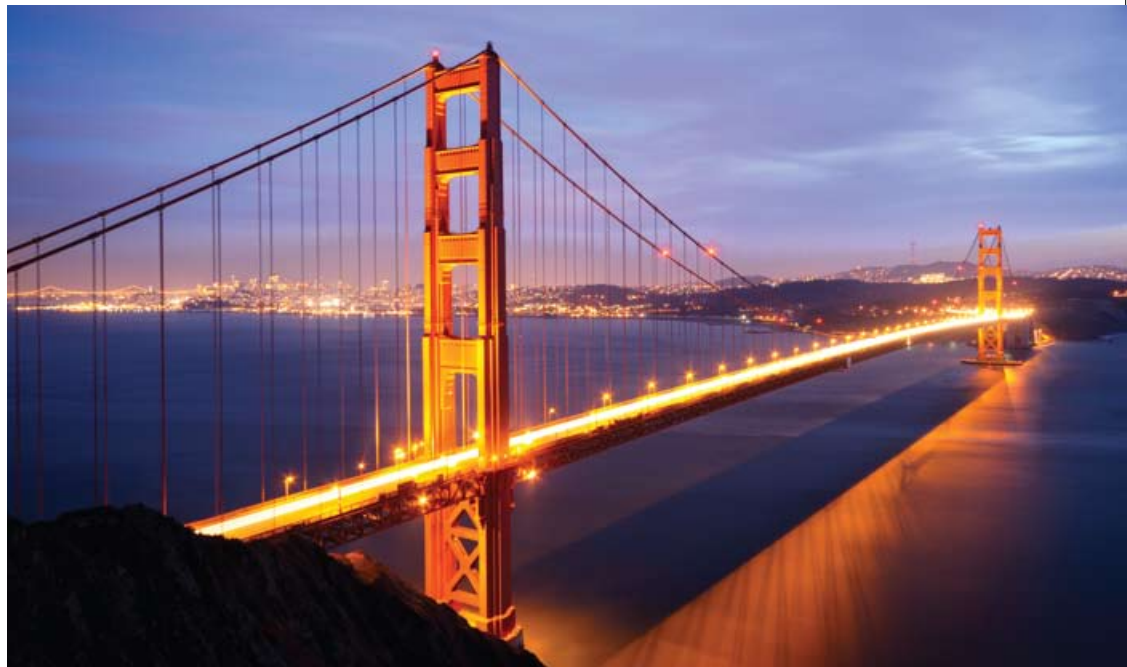
Golden Gate Bridge, San Francisco
