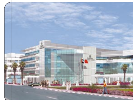
The new Emirates Aviation College.
