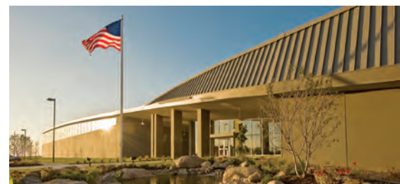
PLATTE WEST WATER TREATMENT PLANT
