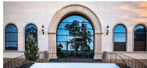
FLORENCE WATER TREATMENT PLANT
